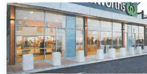
ALUMINIUM-FRAMED CLEAR GLAZING AND GLAZED DOORS. CAPRAL 'ST KILDA' SUITE 150MM POWDERCOAT FINISH. GLAZING SELECTION SUBJECT TO SECTION J
