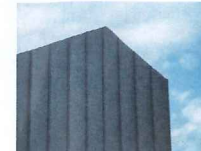
METAL CLADDING - LYSAGHT IMPERIAL PROFILE (USED AS VERTICAL WALL CLADDING. RIBS @ 45 DEGREES) COLORBOND FINISH. COLOUR - BASALT FINISH - MATTE
