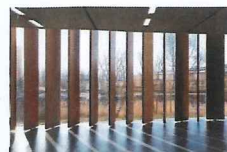
EXTRUDED ALUMINIUM BLADE NOMINALLY 20 X 190 MM @ 450MM CENTRES ALUMINIUM COMPOSITE PANEL - VITRABOND FR CLADDING IN 'BRUSHED COPPER' COLOUR
