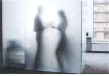
ALUMINIUM-FRAMED OBSCURE GLAZING - AVERY DENNISON DS 1 FILM
