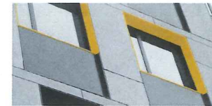
ALUMINIUM WINDOW FRAMES - YELLOW FEATURE COLOUR (TBC) POWDERCOAT GLASS - TO SECTION J REQUIREMENTS
