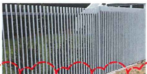
FABRICATED ALUMINIUM TUBE FENCE - SEE DETAILS POWDERCOAT FINISH - YELLOW COLOUR (TBC) AND MID GREY COLOUR (TBC)
