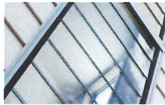
ALUMINIUM-FRAMED CLEAR GLAZING AND GLAZED DOORS. CAPRAL 'ST KILDA' SUITE 150MM POWDERCOAT FINISH. GLAZING SELECTION SUBJECT TO SECTION J
