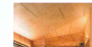
MARINE PLY SOFFIT - POLYURETHANE FINISH. 10MM SHADOWLINE JOINTS EXPOSED COUNTERSUNK GALVANISED FIXINGS
