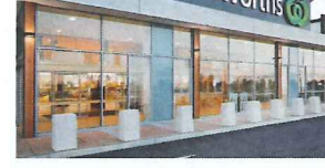
ALUMINIUM-FRAMED CLEAR GLAZING AND GLAZED DOORS. CAPRAL 'ST KILDA' SUITE 150MM POWDERCOAT FINISH. GLAZING SELECTION SUBJECT TO SECTION J
