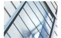
ALUMINIUM-FRAMED CLEAR GLAZING AND GLAZED DOORS. CAPRAL 'ST KILDA' SUITE 150MM POWDERCOAT FINISH. GLAZING SELECTION SUBJECT TO SECTION J
