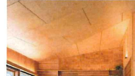
MARINE PLY SOFFIT - POLYURETHANE FINISH. 10MM SHADOWLINE JOINTS EXPOSED COUNTERSUNK GALVANISED FIXINGS
